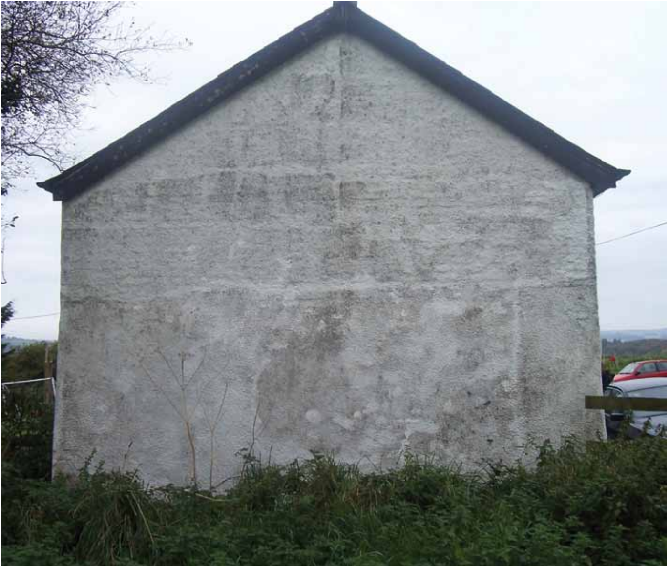
LEFT: Restored to its former glory with lime mortar. ABOVE: This cement render applied to stone and cob shows signs of decay. BELOW: Surveys can pick up problems like this.
