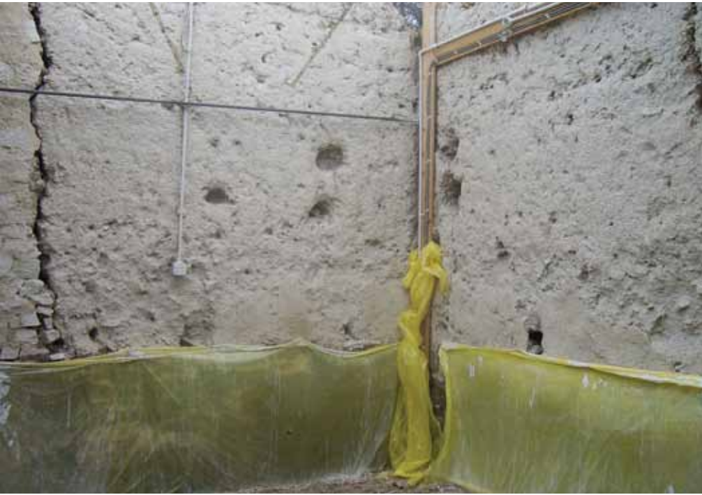
ABOVE: Had a Chartered Surveyor been called in, the cracks in the cob would have been picked up. BELOW: An independent survey would have shown up the shortcomings on this property.
