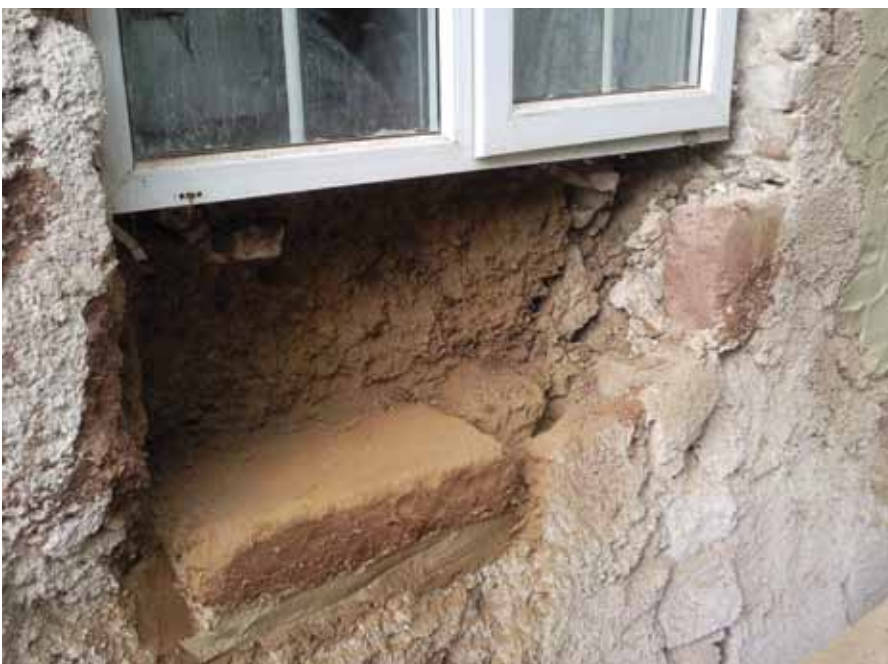
LEFT: Restored to its former glory with lime mortar. ABOVE: This cement render applied to stone and cob shows signs of decay. BELOW: Surveys can pick up problems like this.
