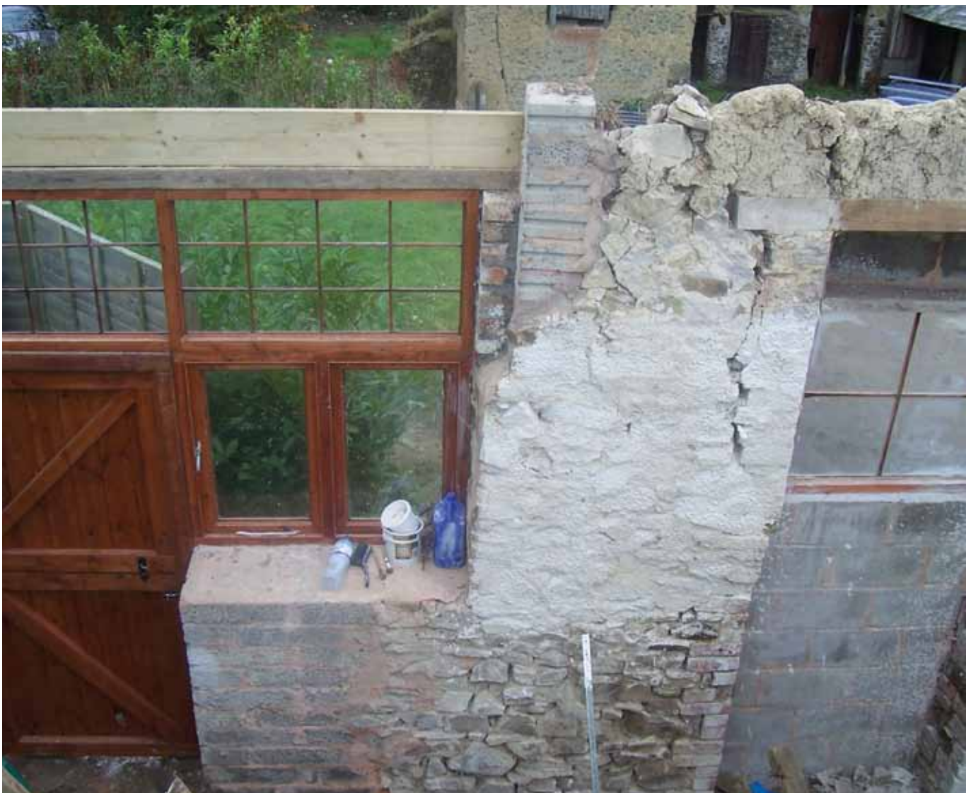
ABOVE: Had a Chartered Surveyor been called in, the cracks in the cob would have been picked up. BELOW: An independent survey would have shown up the shortcomings on this property.
