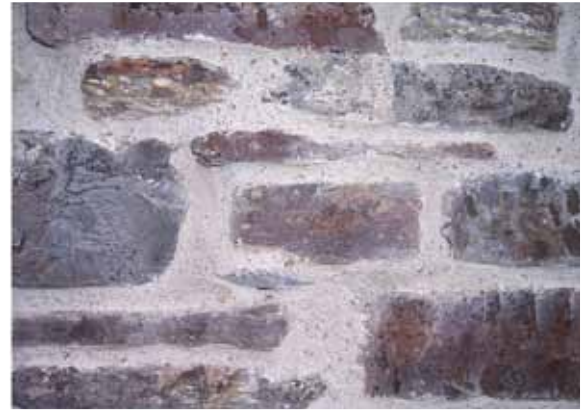
ABOVE CENTER: Cement render before being repointed with lime mortar- notice the cracks that have appeared.
