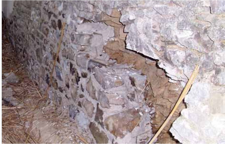
ABOVE: Early stages of restoring decayed stonework.
