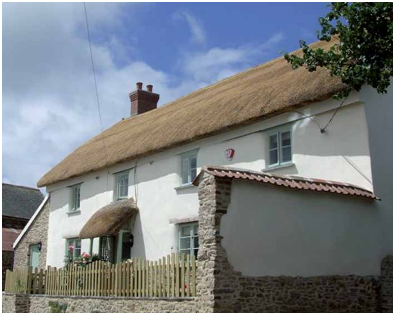
ABOVE: Stone wall and building after restoration.
