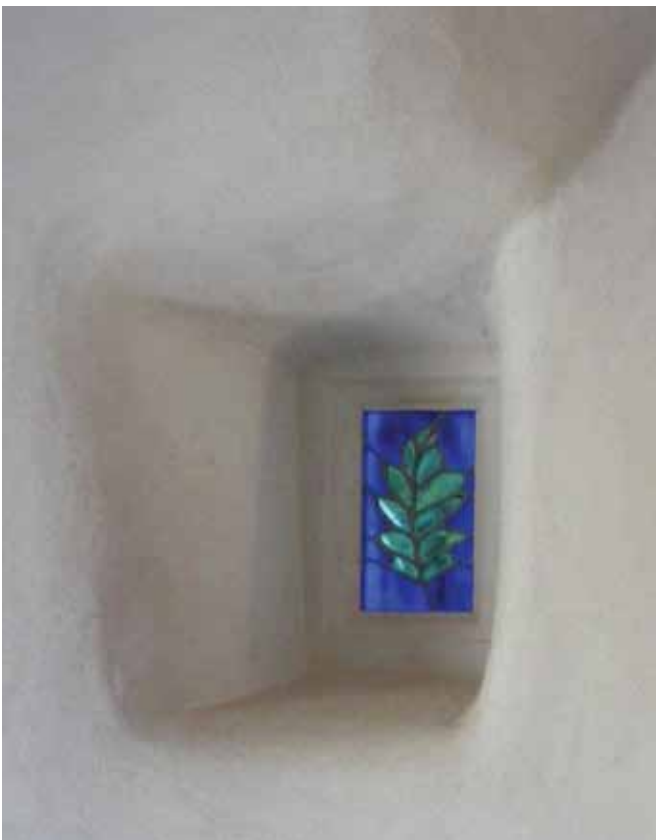
ABOVE: Cobbling around well cover, pillar re-pointed with lime mortar, and steps now in situ. BELOW LEFT: Stain glass window in place- walls rendered with lime mortar. BELOW RIGHT: Wall in annexe lime rendered, leaving feature of window and beam showing
