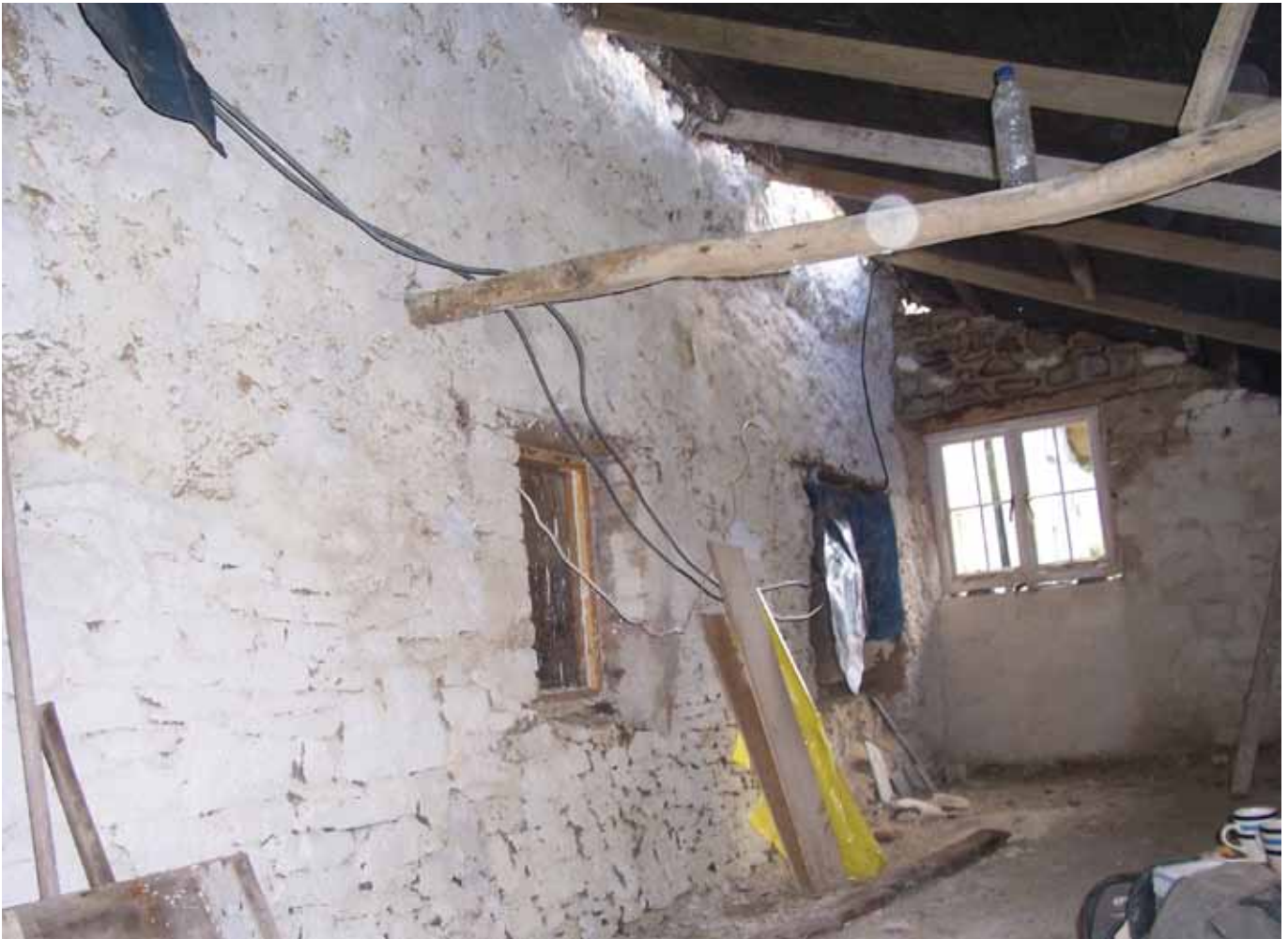
ABOVE: Scat coat on wall of lean to, end wall stoned up and new window in place. BELOW: Close up of stonework near back door- the letter F was engraved in the original stone.
