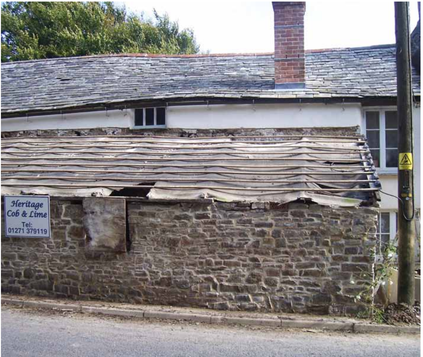
LEFT: Windows in place, stone work re-pointed with lime mortar. ABOVE: Slates are off, roof awaiting repair. BELOW: The well- it looks small but goes down 30 feet and turned out to be 6 feet in diameter.
