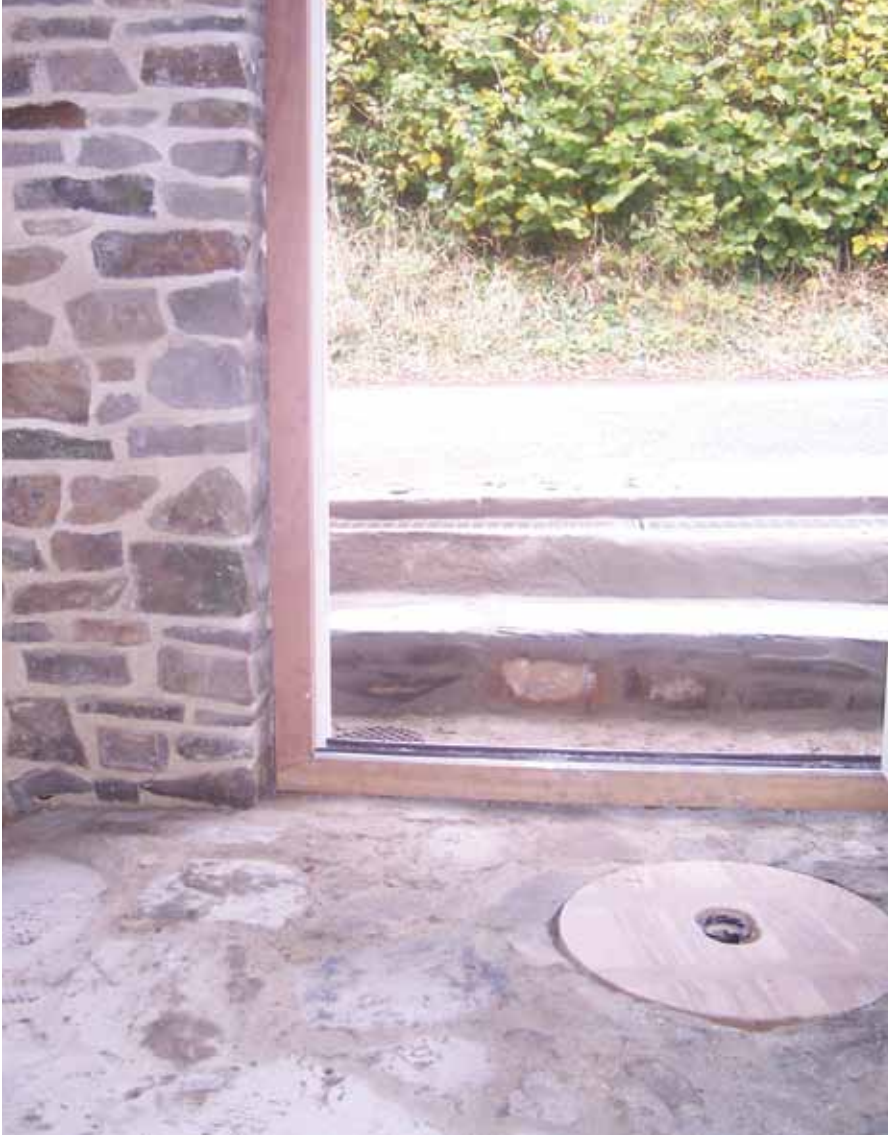
ABOVE: Cobbling around well cover, pillar re-pointed with lime mortar, and steps now in situ. BELOW LEFT: Stain glass window in place- walls rendered with lime mortar. BELOW RIGHT: Wall in annexe lime rendered, leaving feature of window and beam showing
