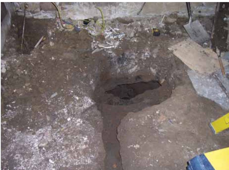
LEFT: Windows in place, stone work re-pointed with lime mortar. ABOVE: Slates are off, roof awaiting repair. BELOW: The well- it looks small but goes down 30 feet and turned out to be 6 feet in diameter.
