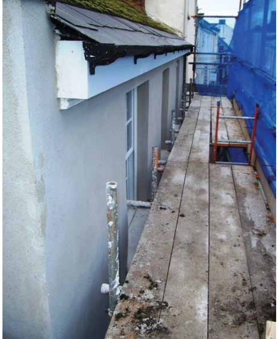
ABOVE: Lime render now ready for limewashing on this listed property in Bideford, North Devon. BELOW: Final coat, limewashed in Marigold, property circa 1930
