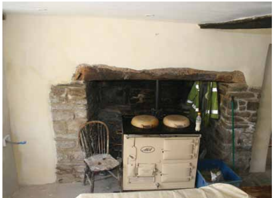
LEFT: Applying a scratch coat to this 1930's property. ABOVE: Newly applied lime mortar, that's still drying out. BELOW LEFT: Before starting work on this barn conversion, circa 1700. BELOW: A top coat of lime render has been used on the exterior of this barn conversion.
